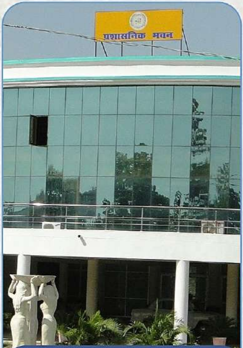
Administrative Building ANDUA&T, Ayodhya
